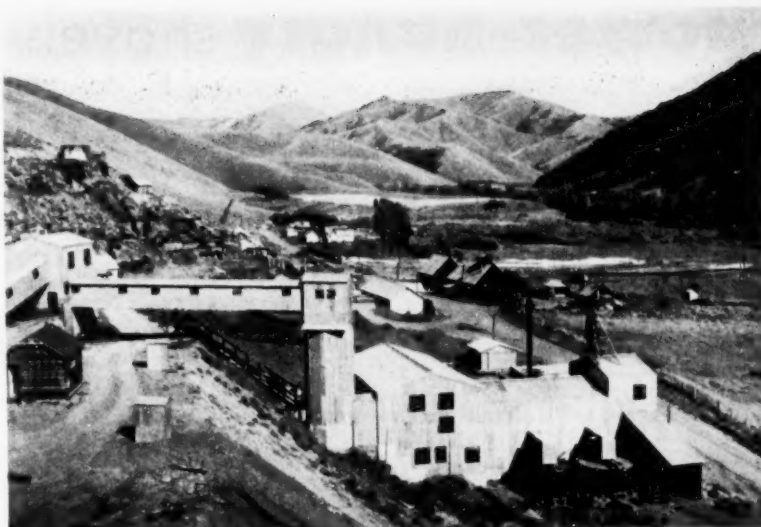
The 300 ton per day selective flotation mill of the Triumph Mining Company was placed in operation in 1951. It is one of the most modern and efficient in the United States.
